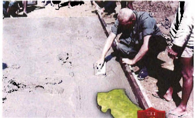
Although they were not supposed to do the job by themselves, CA personnel had to 'get dirty.' They often had to show the villagers how to perform tasks, get them enthused in a project, and then step back so that they developed a sense of ownership.
